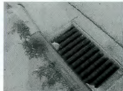
Untreated stormwater entering a storm drain.
